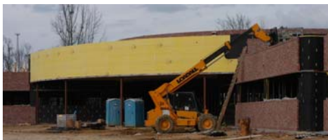
Construction of the 40,000 sq. ft. Literacy and Technology Center
